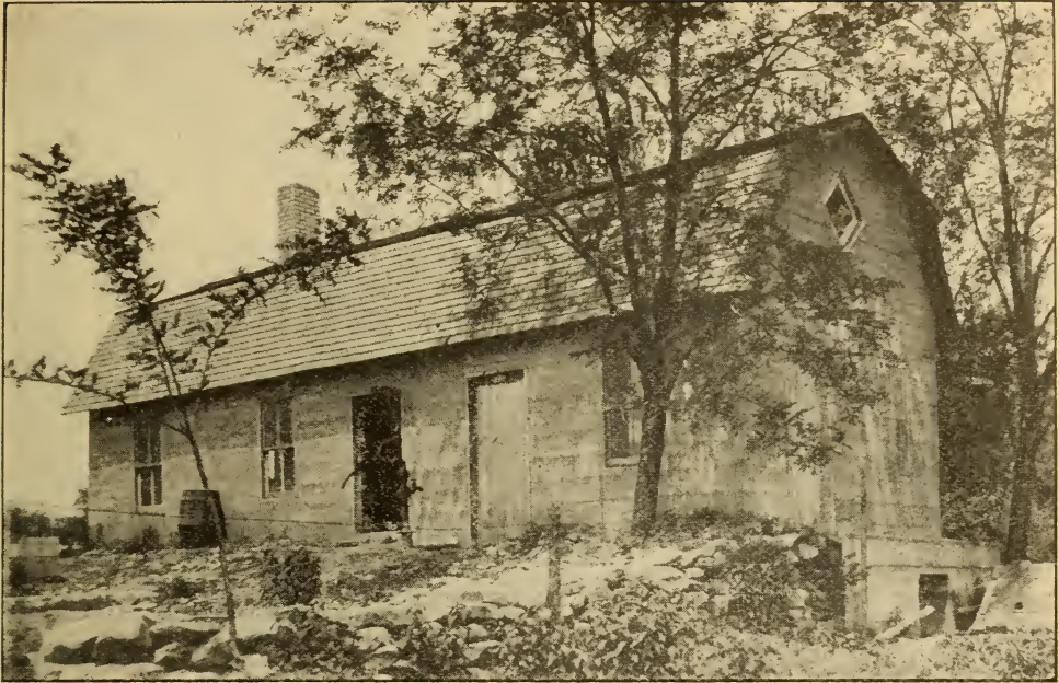
David Running's 16 x 40-foot concrete building. There are two different floors besides the cellar where the bees are wintered. The cellar has a capacity for nearly 350 colonies. Where gravel is cheap, concrete is cheaper than lumber in the long run.
